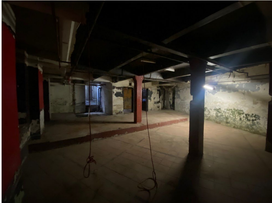
interior - basement level
