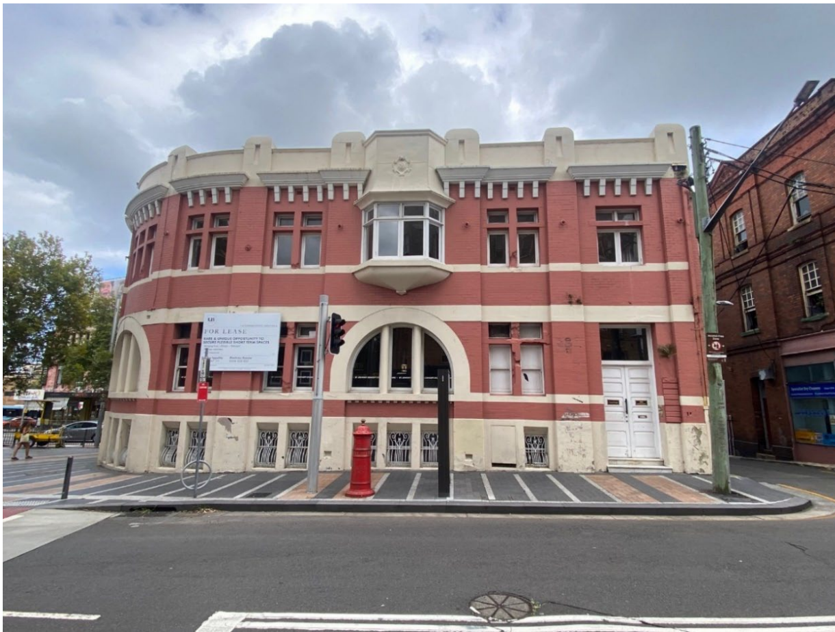
site viewed from Bourke Street
